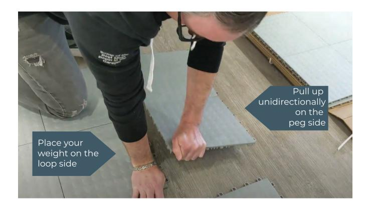
It is very important to only pull up on the peg side. If you pull up on the loop side you can break the loops.
